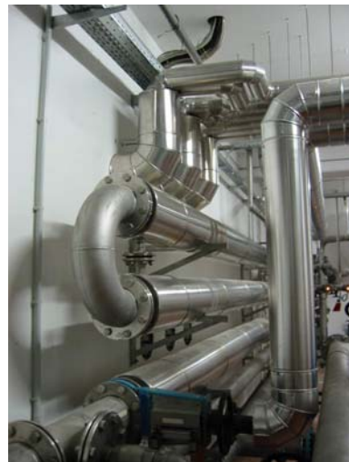
Sludge Heat Exchangers
