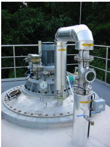
Gas Hood for draft tube mixer installation
